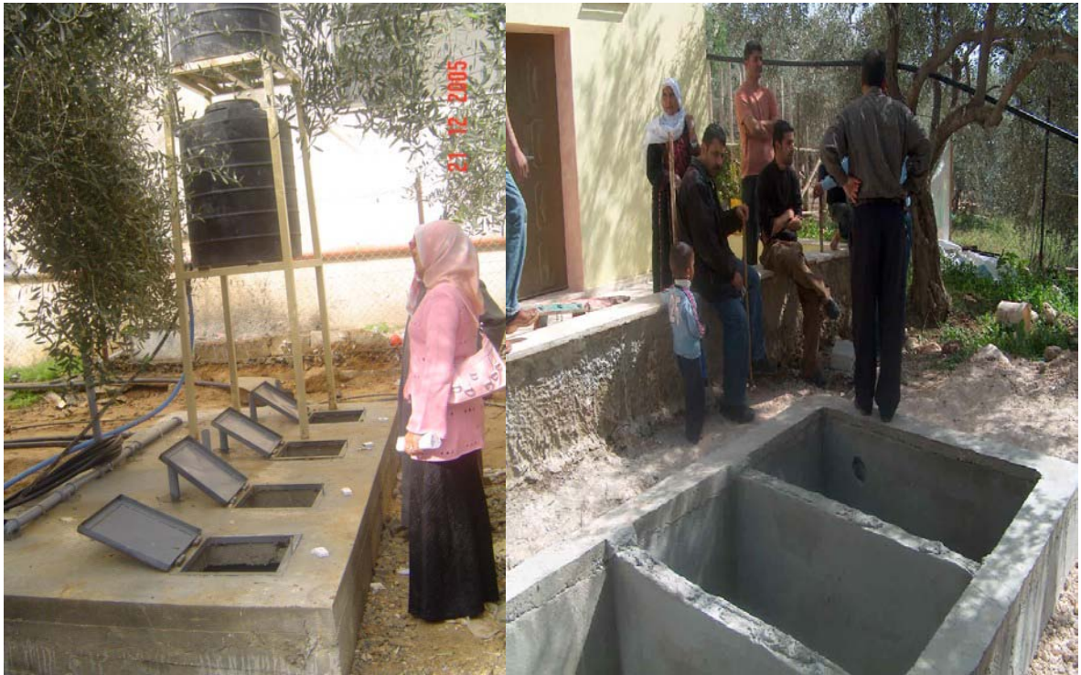
Figure (2): GWWTPs projects implemented by PHG in Gaza Strip.
