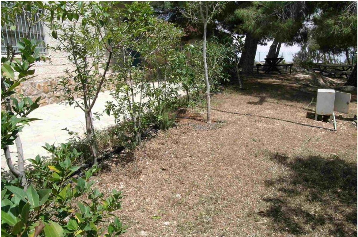
Photo 5.Example of a drip irrigation system using reclaimed water from the ARIJ process
