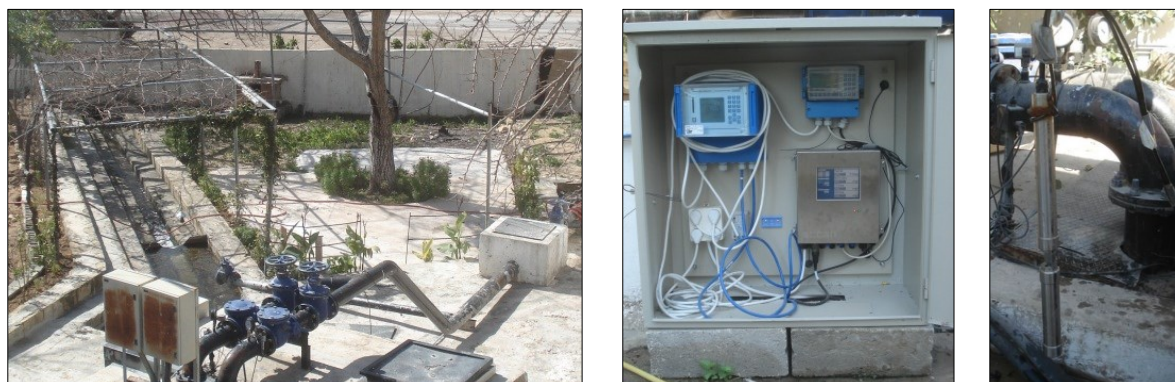
Figure 28: Fotos of Hazzir Spring (left) and monitoring devices. Box with monitoring devices (middle) and UV-Vis probe (right).
