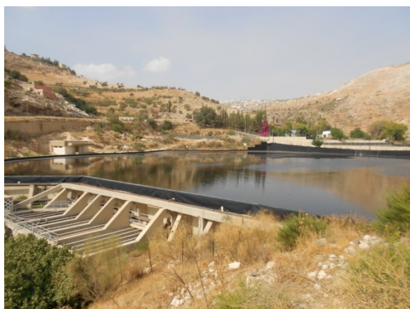
Figure 13: Maturation pond of As Salt WWTP (Zemann, 2012)
