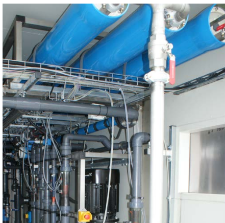
Figure 9: Reverse Osmosis unit (photo: SPA).
