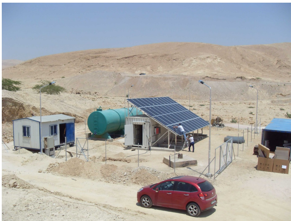
Figure 11: Installation of solar plant in Karameh (photos: SPA).
