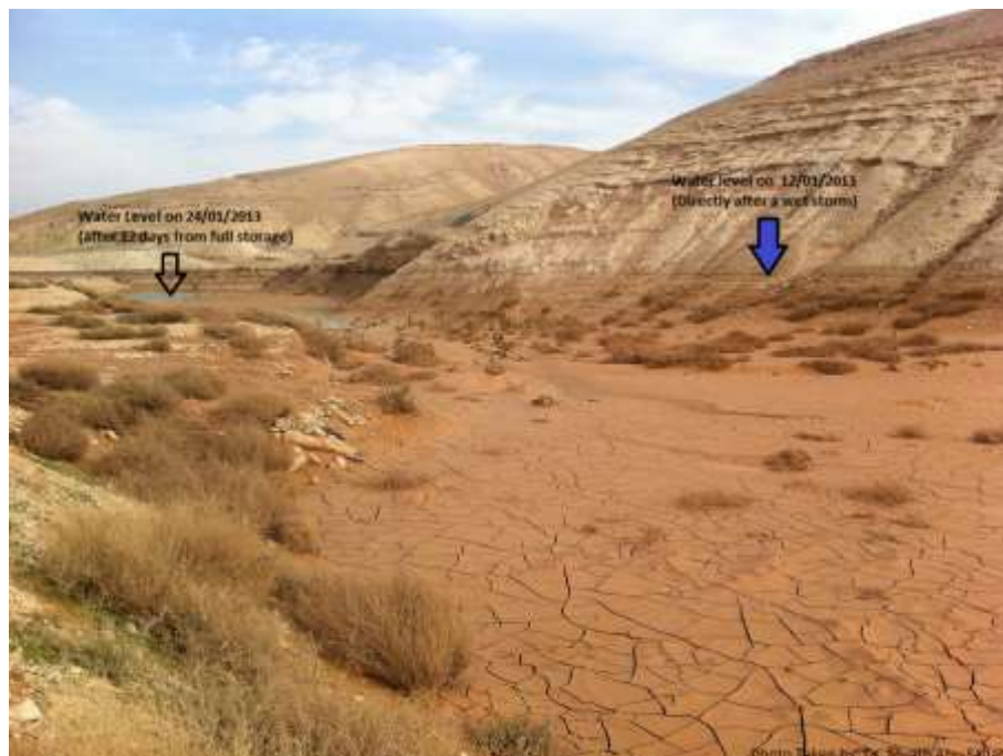
Figure 4.9: Auja surface reservoir on January 24th 2013. The arrows show the strong reservoir depletion after a rainfall-runoff event due to infiltration losses (photo: Muath Abu Sadah, HEC).
