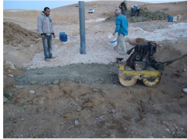
Fig.13: Bentonite compaction
