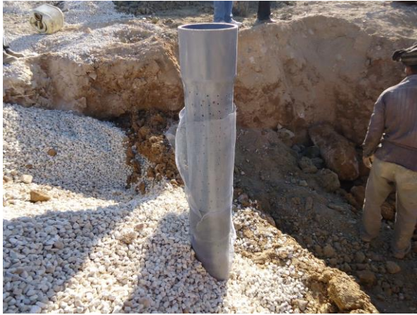
Fig.12.: The pipe installation
