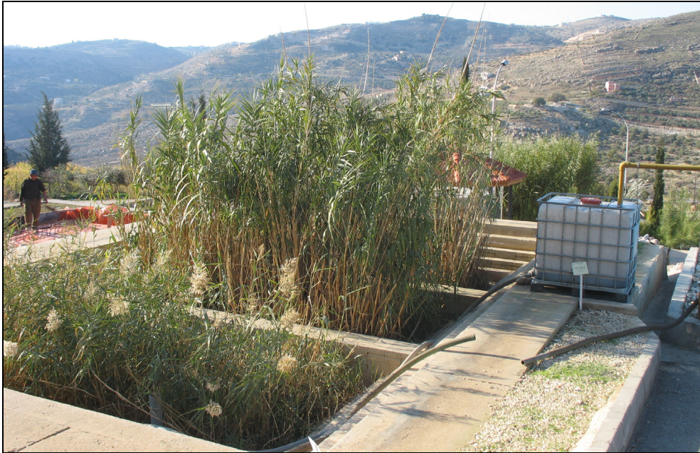
Figure 5: Photo of the three SDRBs which are operating under sludge loading rate at the Fuhais site
