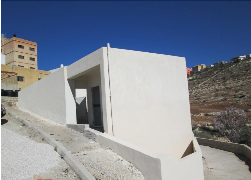
Figure 6: Front side of the new MBR-system building on the site in Maghareeb
