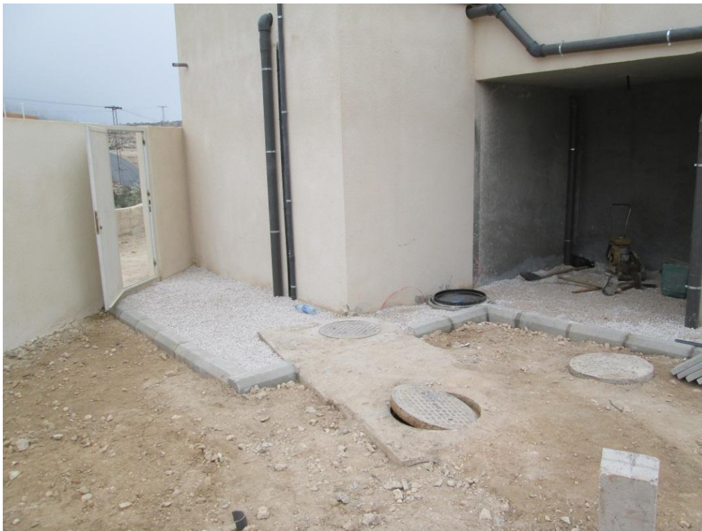
Figure 9: New building implemented around the existing septic tank (see tank covers on the ground)
