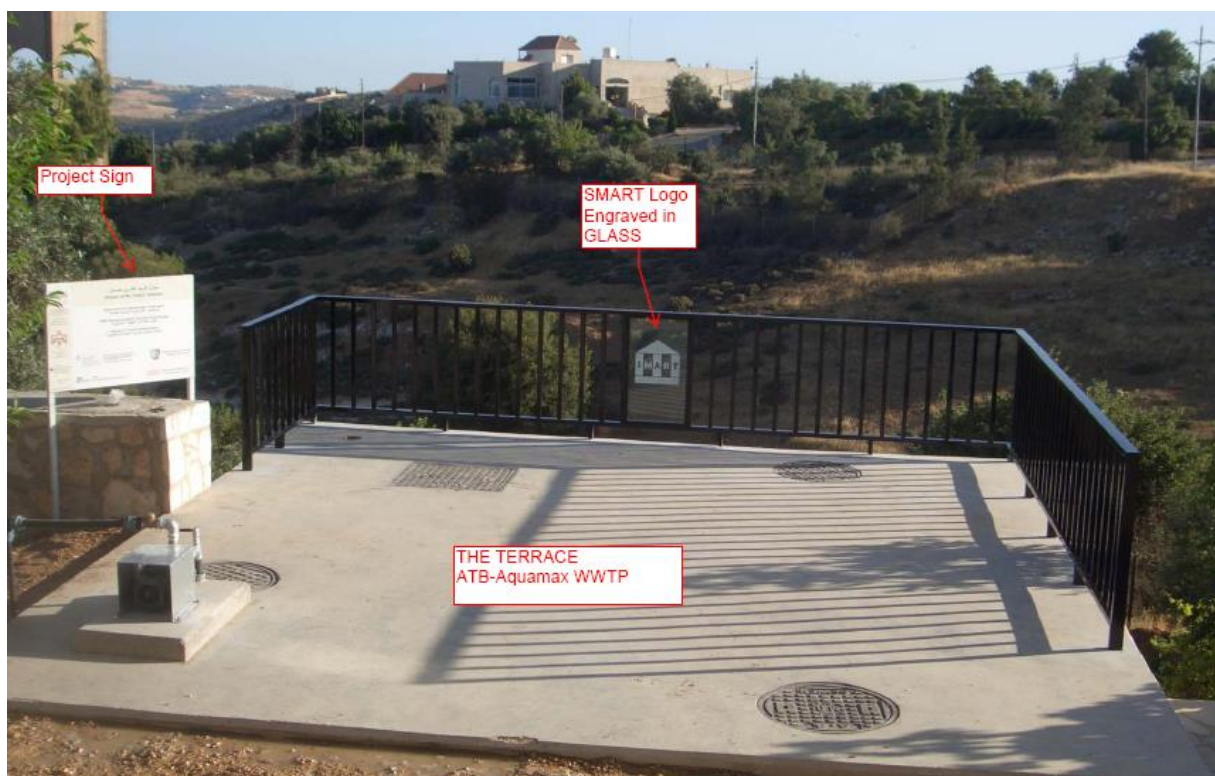
Figure 4: The SBR tank - the Terrace - after completion.
