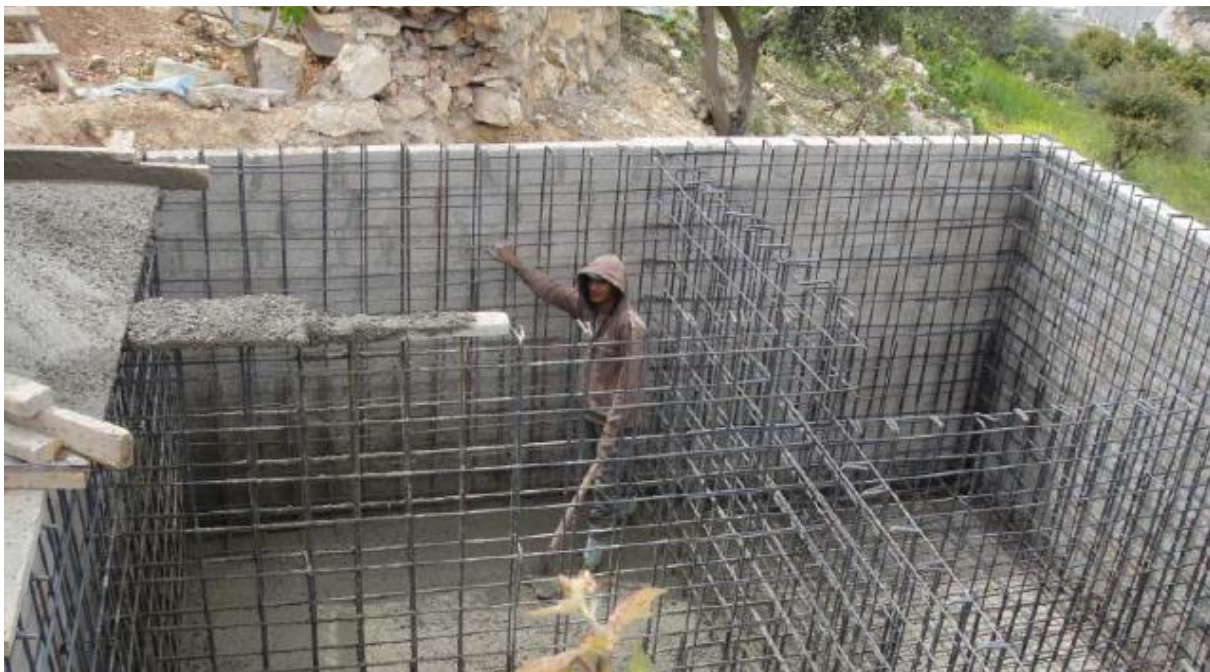
Figure 2: Pouring of the bottom concrete slab of the SBR tank.
