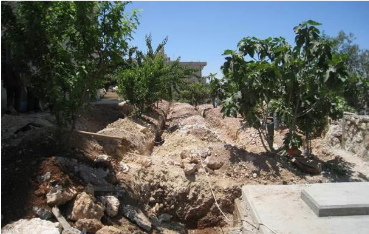
Figure 5: Excavation of the irrigation trench in the upper garden.
