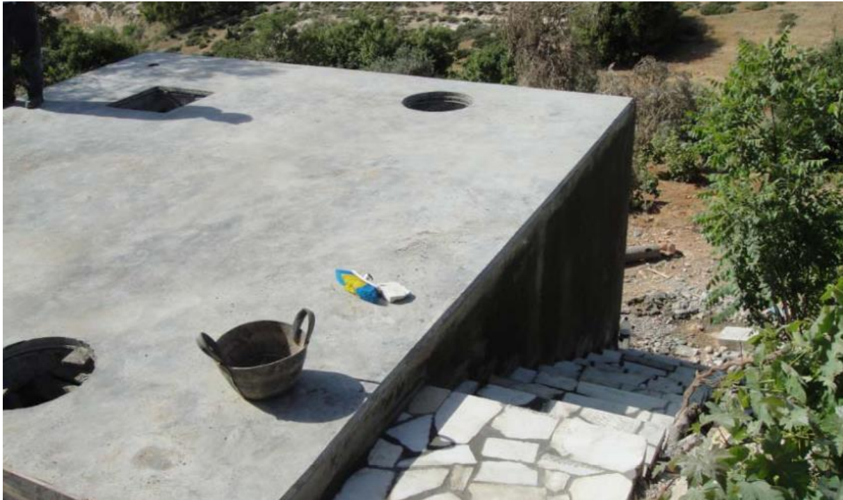
Figure 3: The SBR tank and the stairs after the end of the concrete work.
