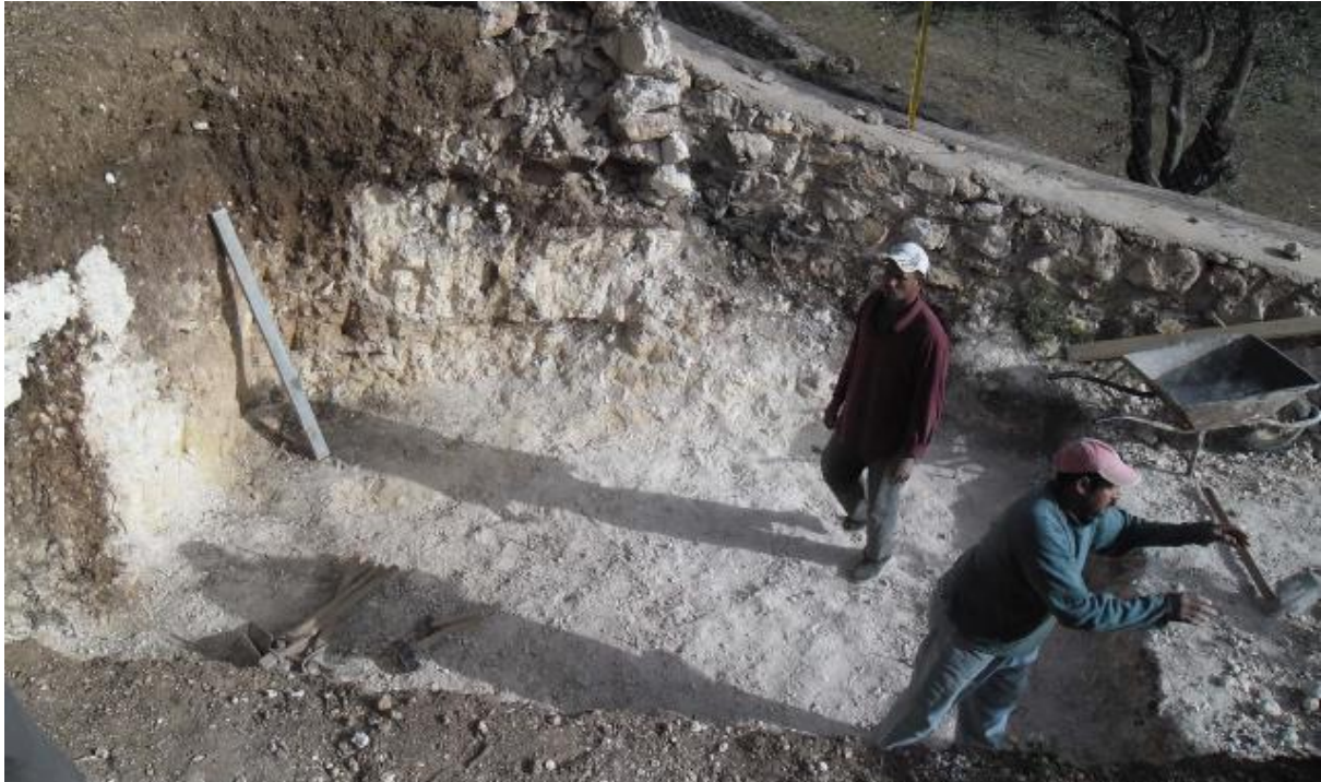
Figure 12: Excavation of the pit for the installation of the SBR tank.
