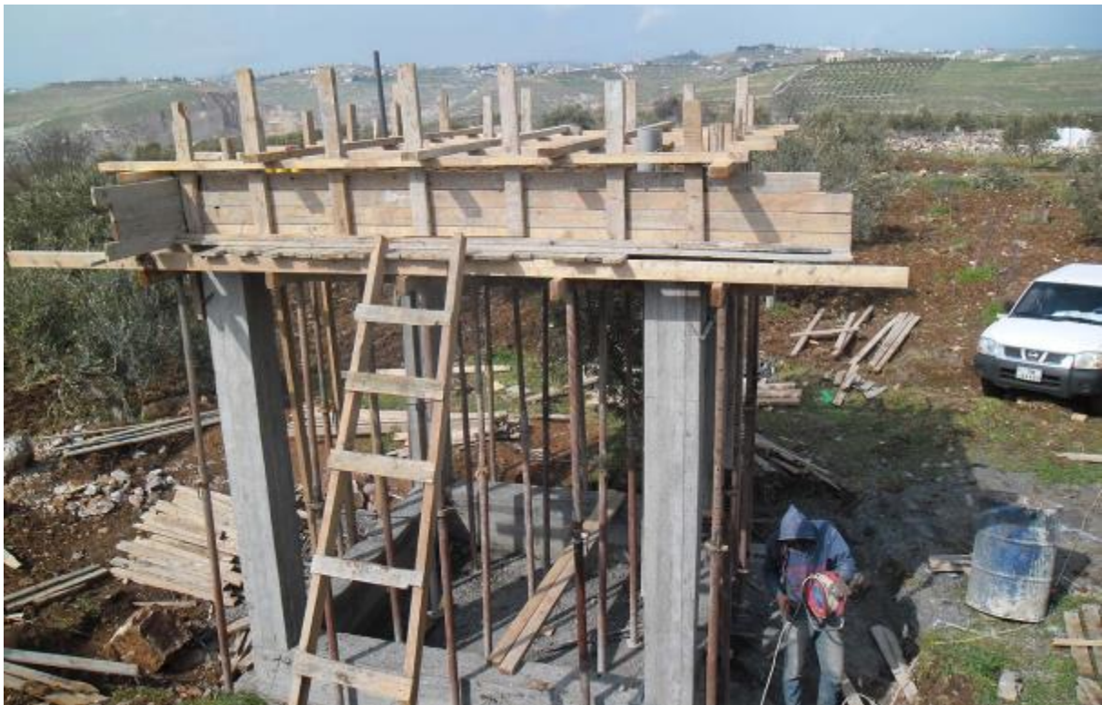
Figure 27: Construction of the water tower in the garden.
