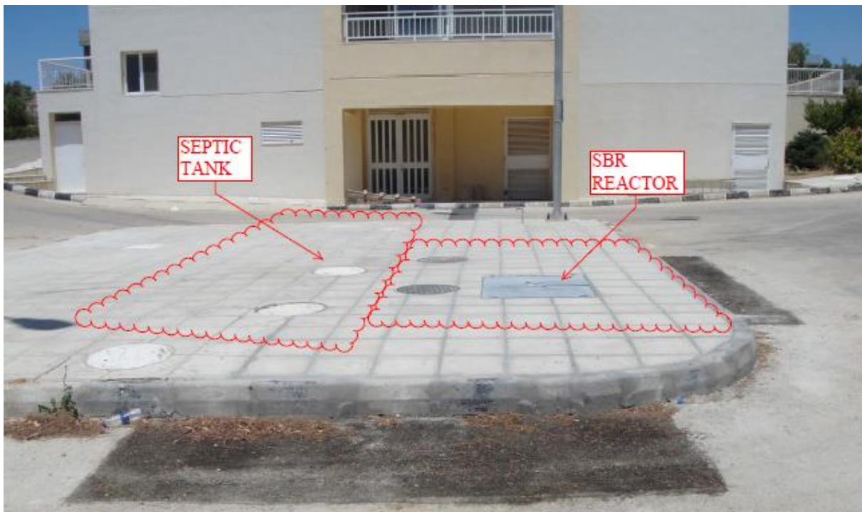
Figure 24: The SBR tank after completion.
