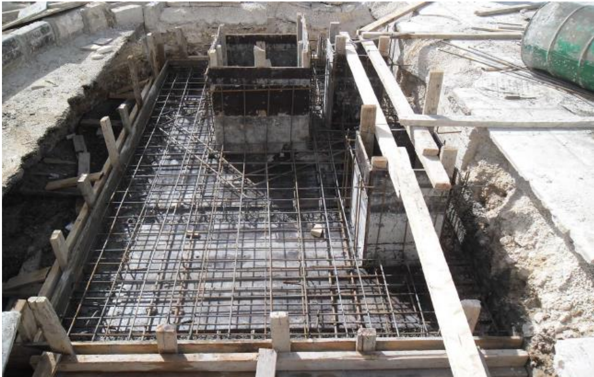
Figure 23: Construction of the top of the SBR tank.
