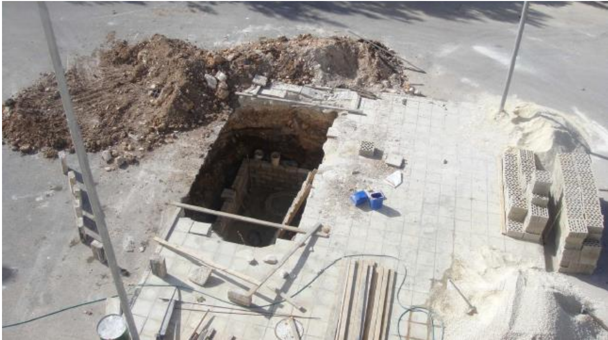
Figure 21: Excavation of the pit for the installation of the SBR tank.
