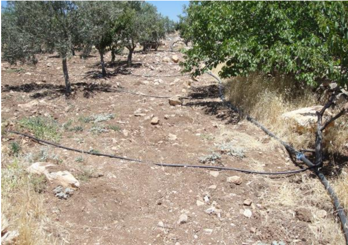
Figure 29: The drip lines installed in the reuse area.
