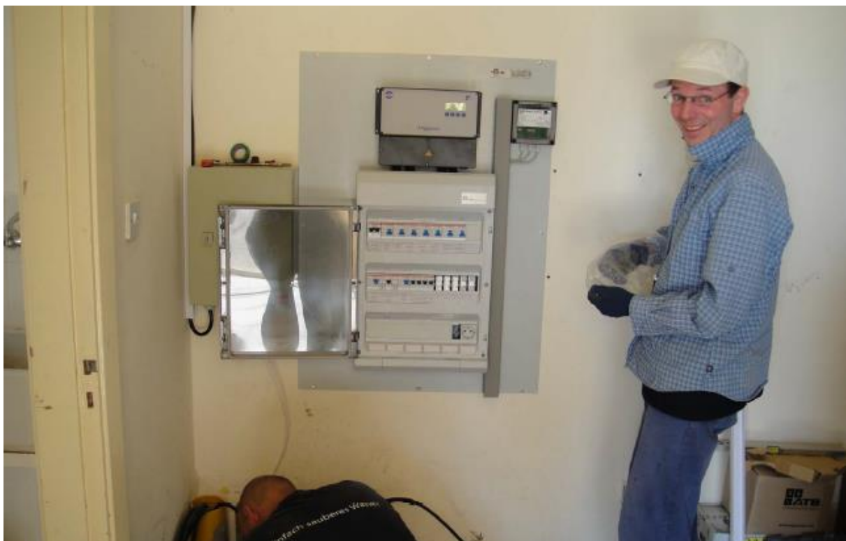
Figure 26: Installation of the control panel to operate the SBR.
