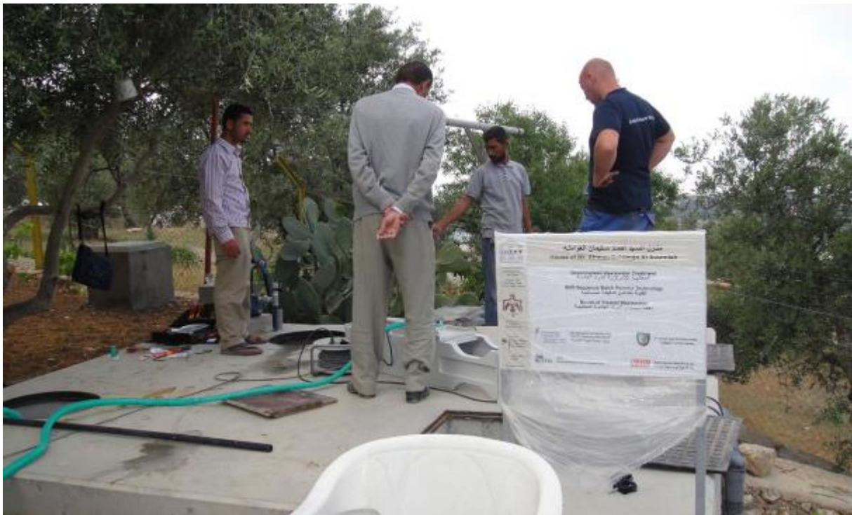
Figure 17: Installation of the SBR unit.
