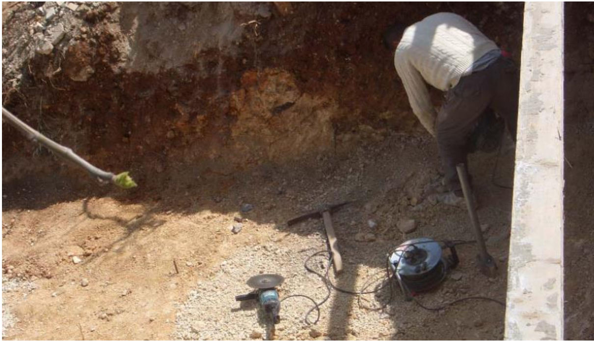
Figure 1: Excavation of the pit for the installation of the SBR tank.
