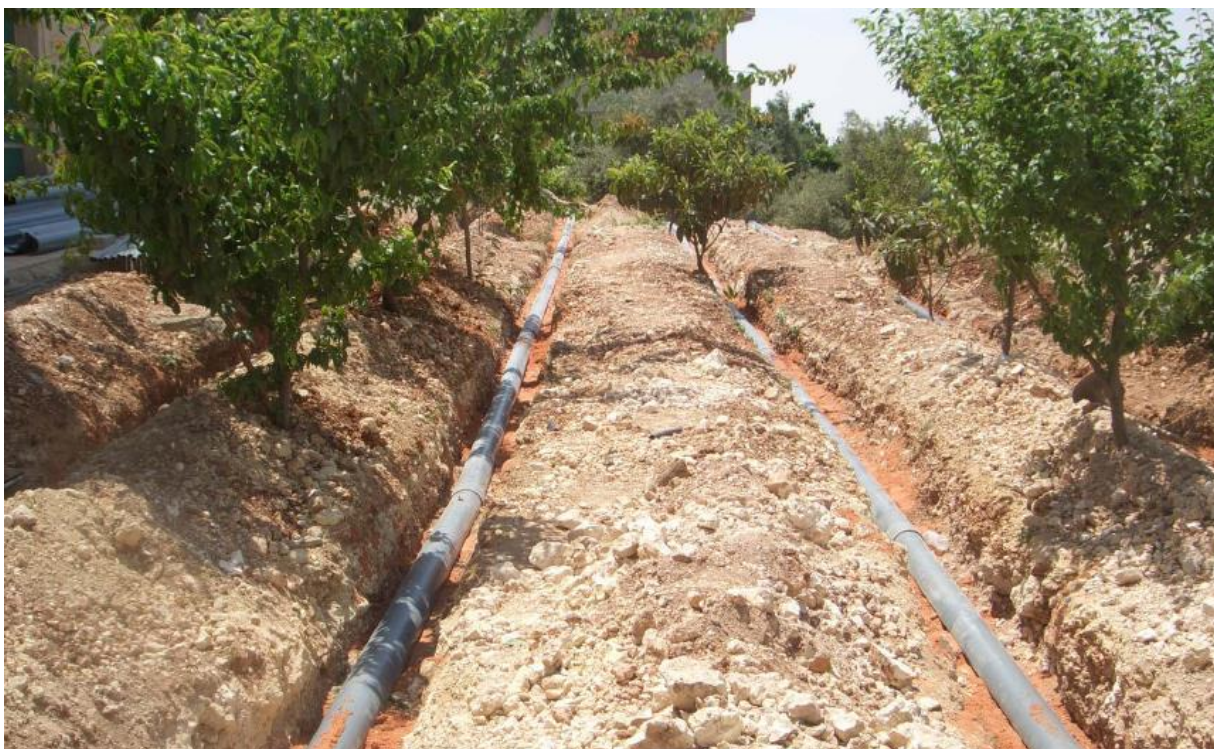
Figure 6: Installation of the subsurface irrigation lines in the upper garden.
