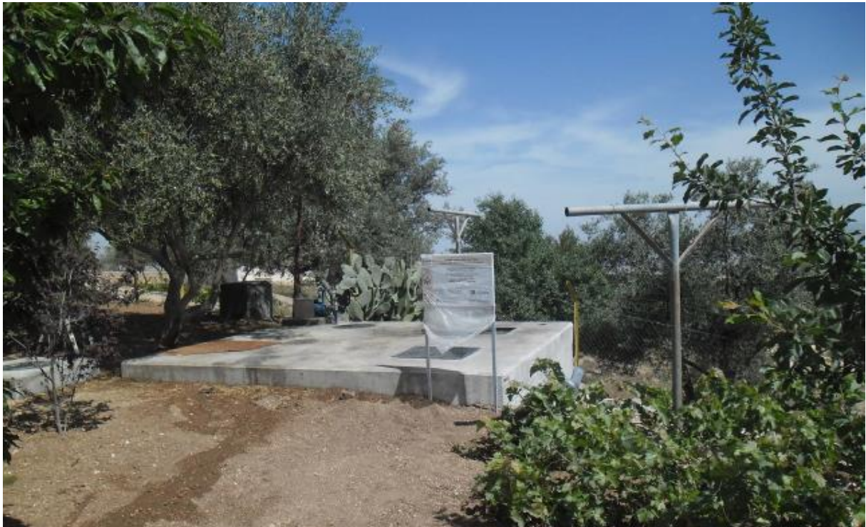
Figure 14: The SBR tank after the end of the concrete work.
