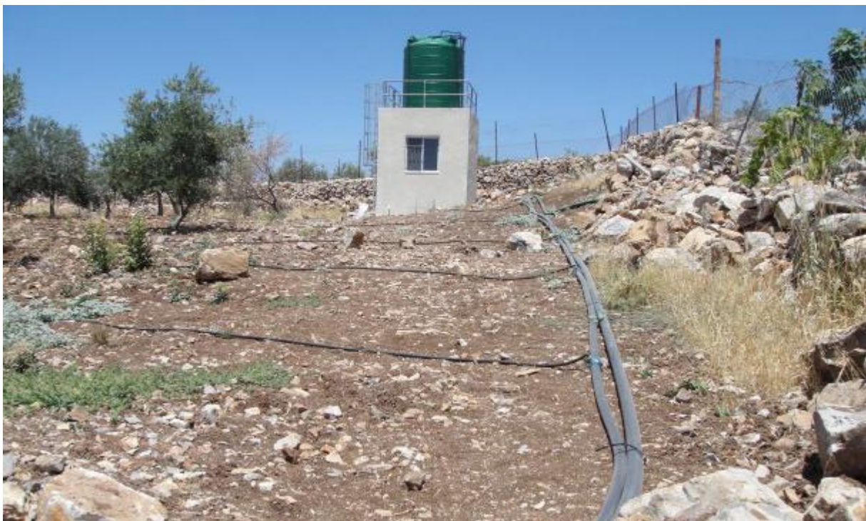
Figure 28: The water tower, its storage room and the drip irrigation lines after completion.
