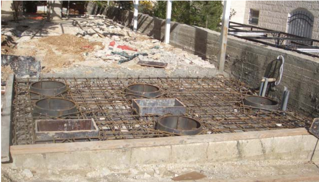
Figure 3: Installation of the manholes and covers.
