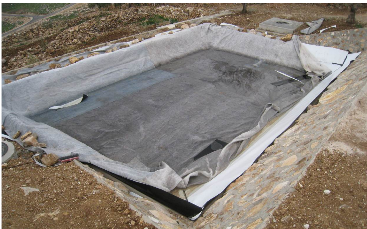
Figure 34: Installation of the liner and geotextile in the wetland.
