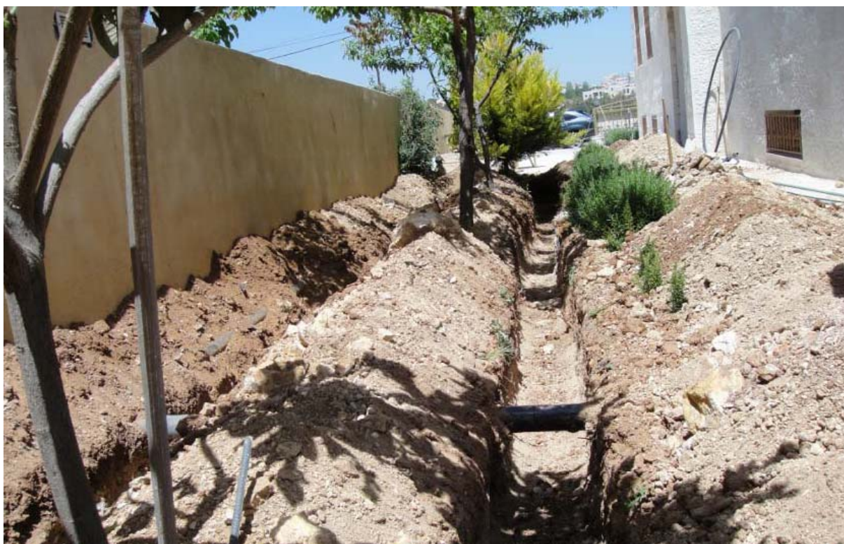
Figure 16: Excavation of the irrigation trenches.
