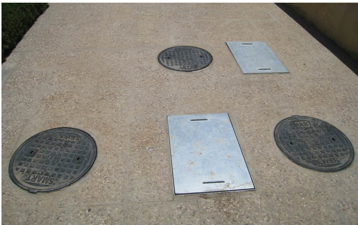
Figure 15: Mr Shehabi's Modified Septic Tank after the end of the construction.
