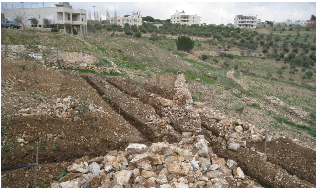
Figure 41: Excavation of the irrigation lines.
