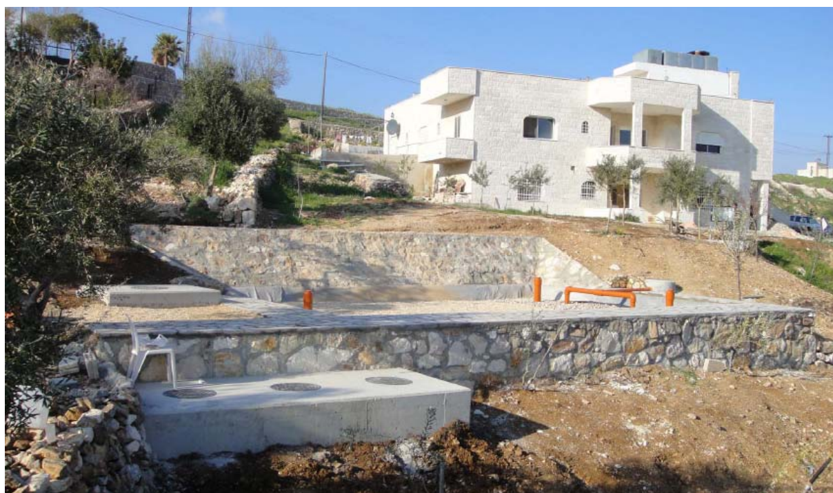
Figure 40: Mr Hadidy's wetland, flow splitting box and irrigation tank after completion.
