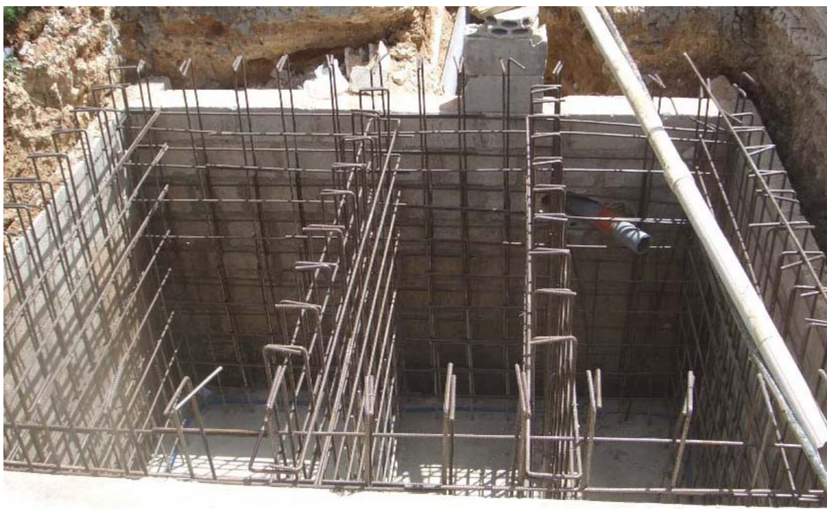
Figure 13: Concrete walls and reinforcing steel of the Modified Septic Tank.
