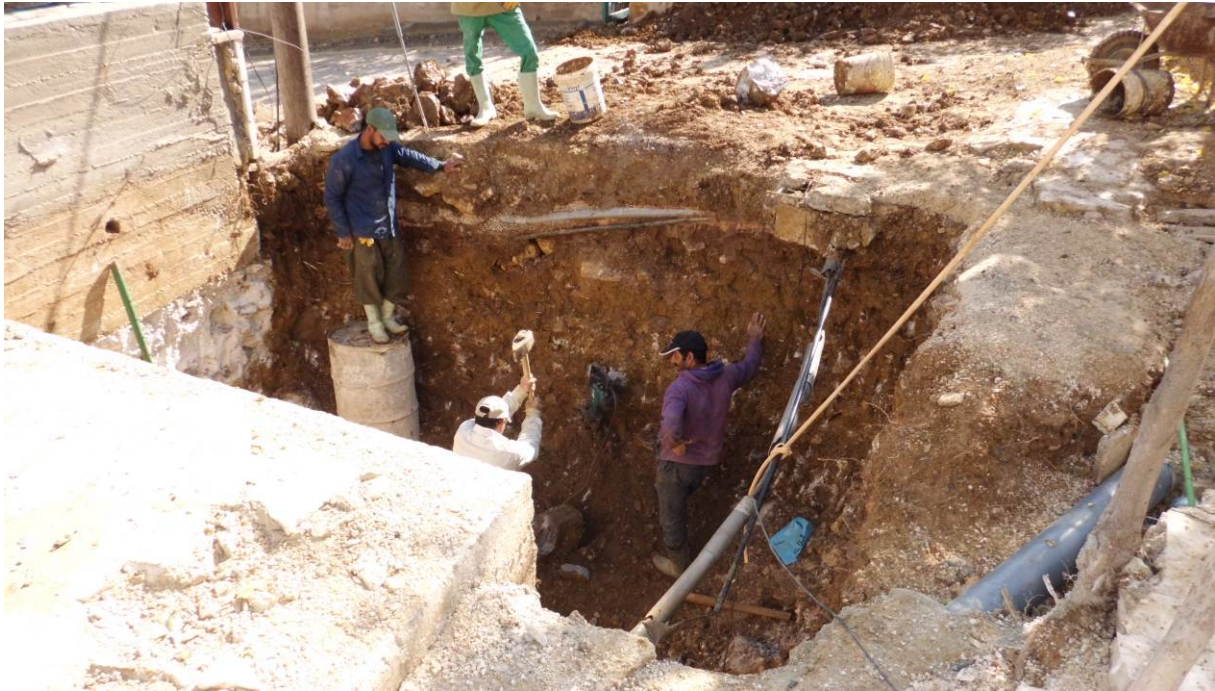
Figure 1: Excavation pit for the Modified Septic Tank
