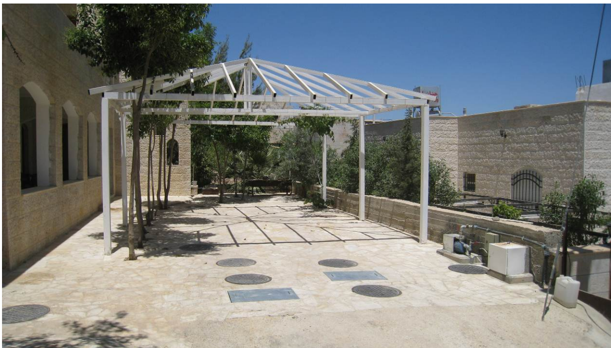
Figure 4: Mr Hiyari's Modified Septic Tank after the end of the construction.
