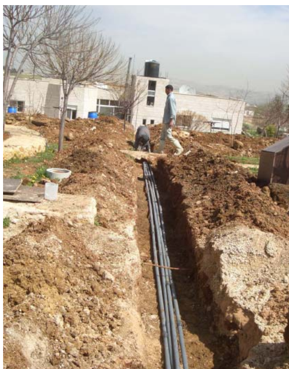
Figure 6: Installation of the irrigation lines in the garden.
