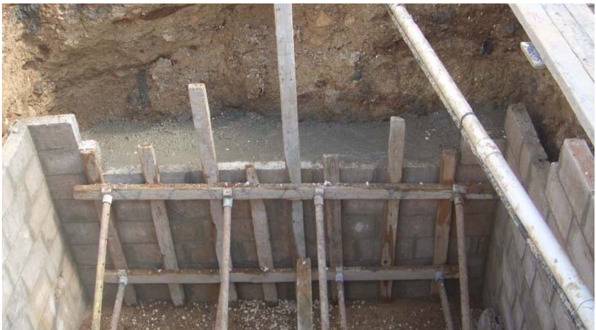
Figure 12: Reparation of the wall collapse.
