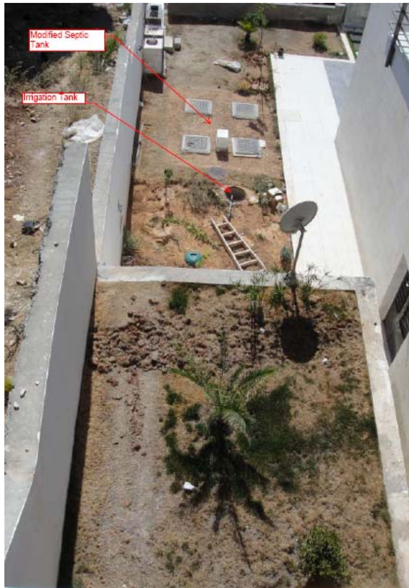
Figure 25: The Modified Septic Tank in Mr Akeel's garden.
