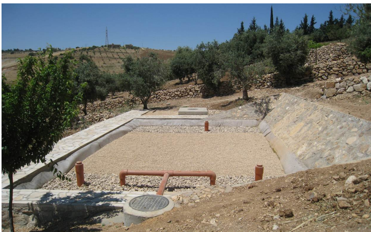
Figure 36: The wetland after completion.
