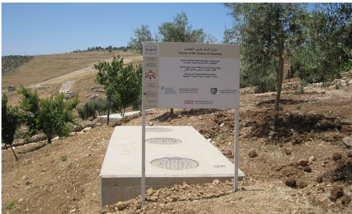
Figure 31: The septic tank after completion.
