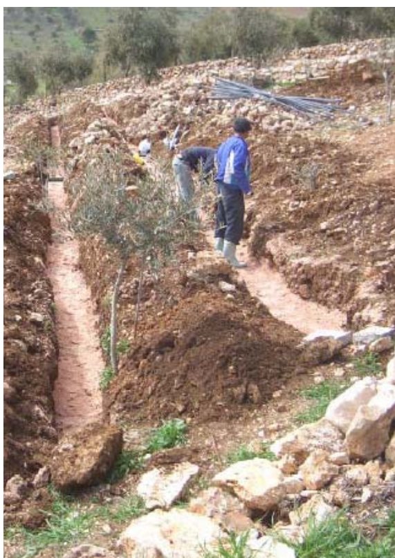
Figure 42: Installation and water testing of the irrigation lines.
