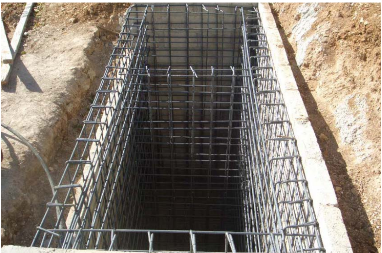
Figure 30: Concrete form and reinforcing steel of the septic tank.
