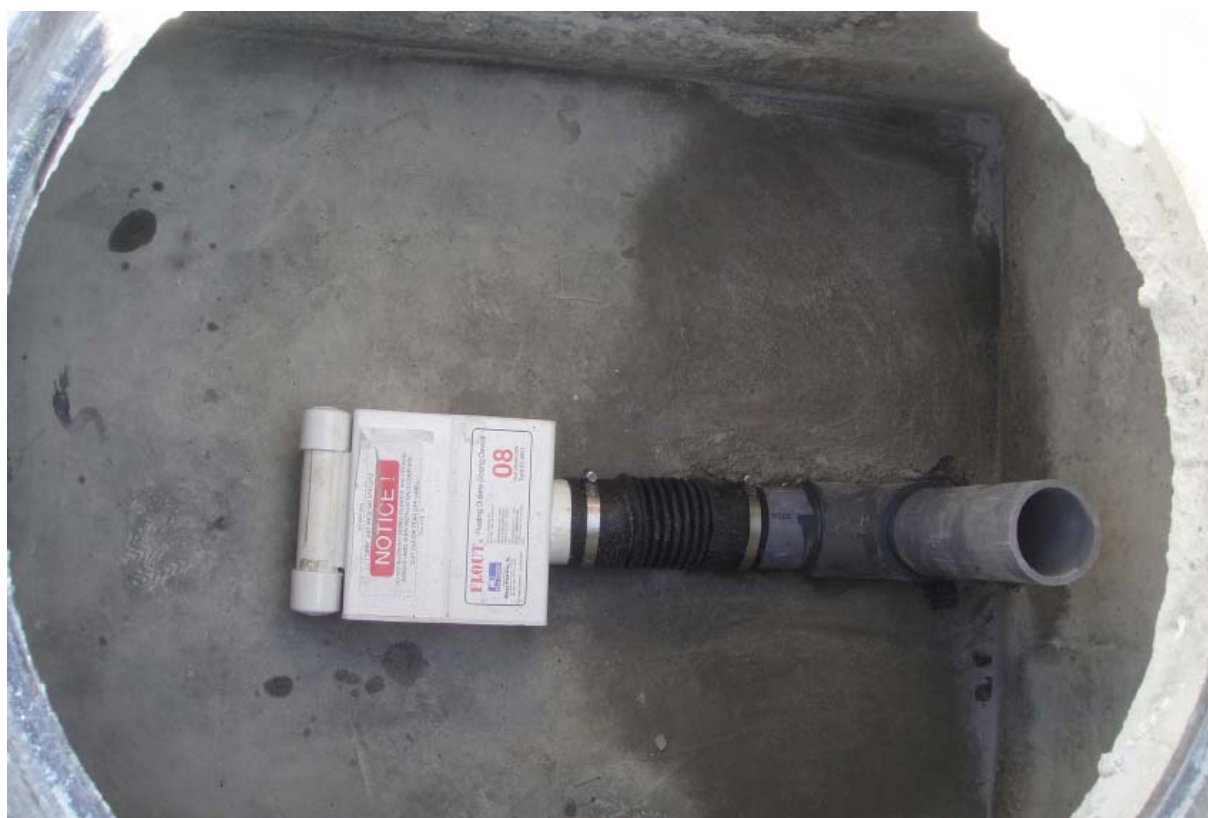
Figure 39: Flow dosing device (flout) for the irrigation fields.
