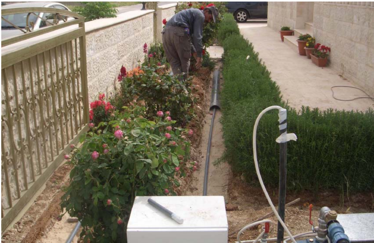
Figure 17: Installation of the irrigation lines in the front yard.
