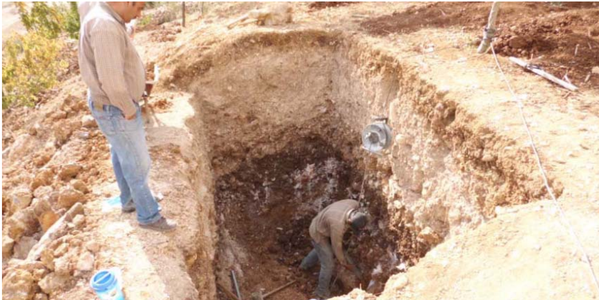
Figure 29: Excavation of the septic tank.
