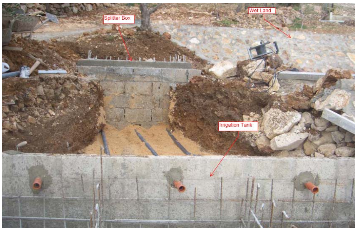
Figure 37: Concrete walls and reinforcing steel of the flow splitting box and irrigation tanks.
