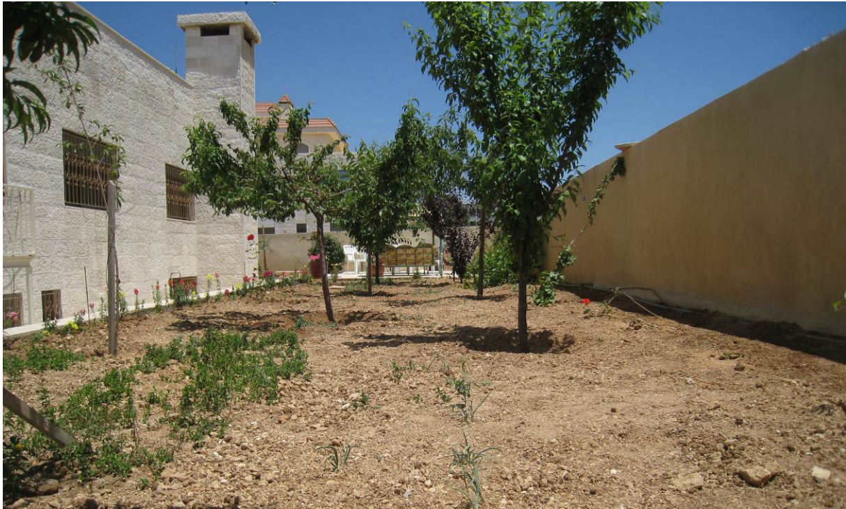
Figure 19 Mr Shehabi' garden after the installation of the irrigation lines.
