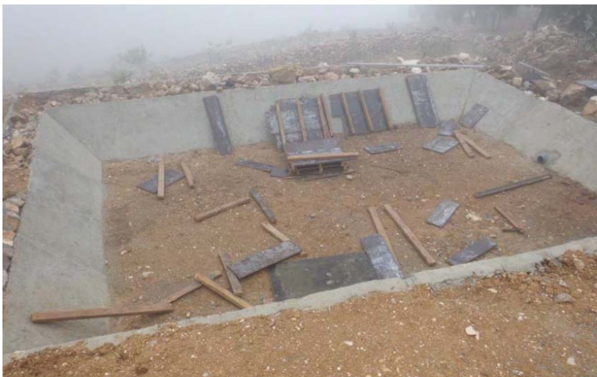
Figure 33: Construction of the wetland.
