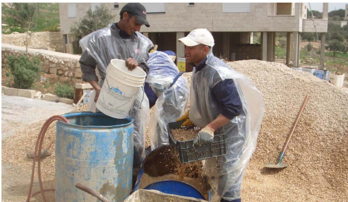
Figure 35: Preparation (cleaning) of the wetland's filter media.
