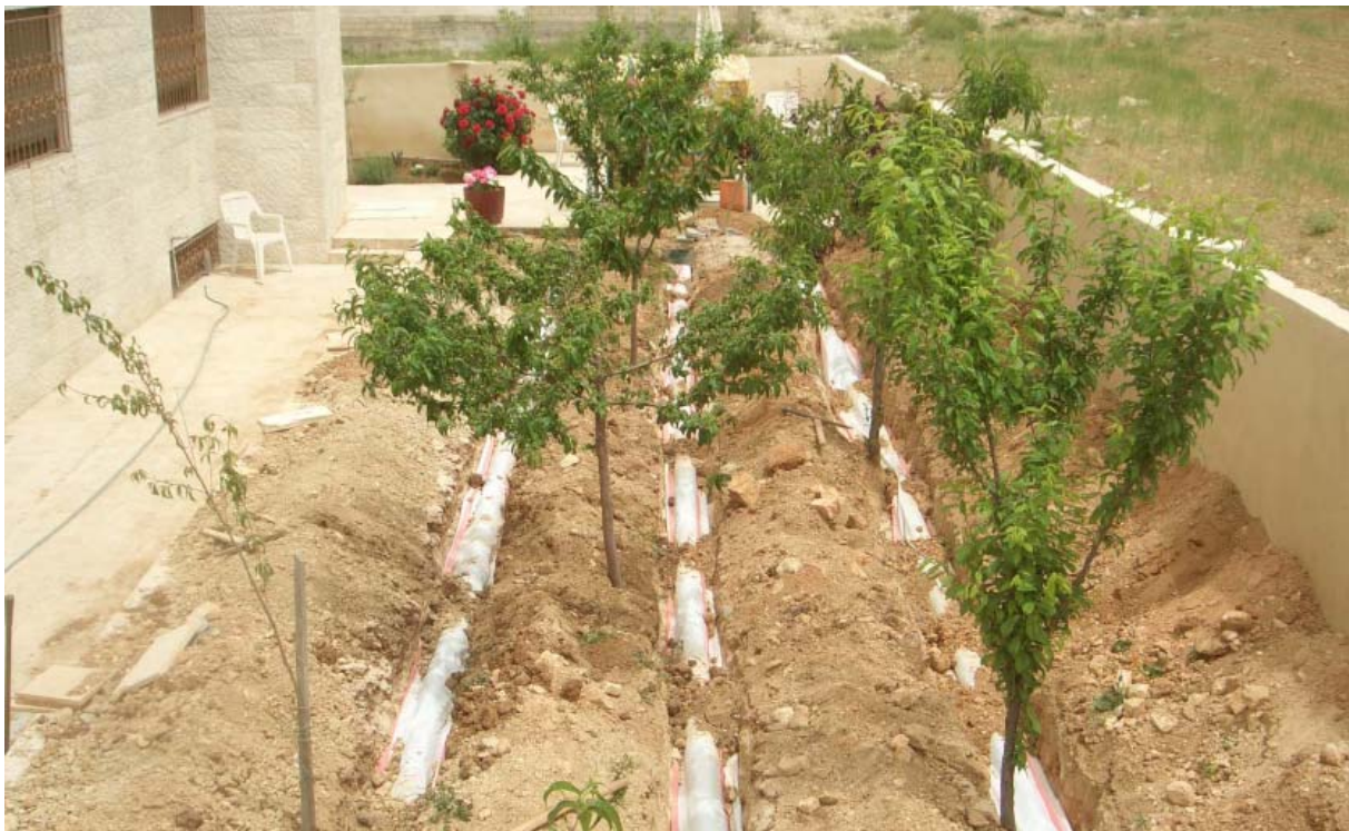
Figure 18: Installation of the irrigation lines in the back yard.
