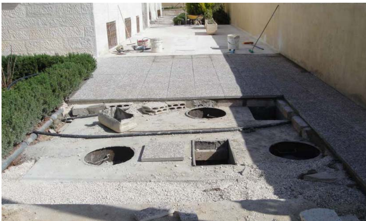
Figure 14: Reinstalment of the tiles.
