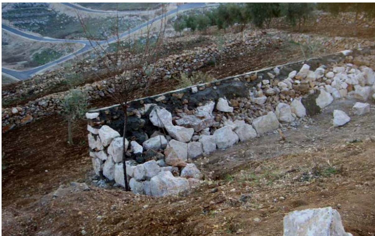
Figure 32: construction of the retaining walls before the installation of the wetland.
