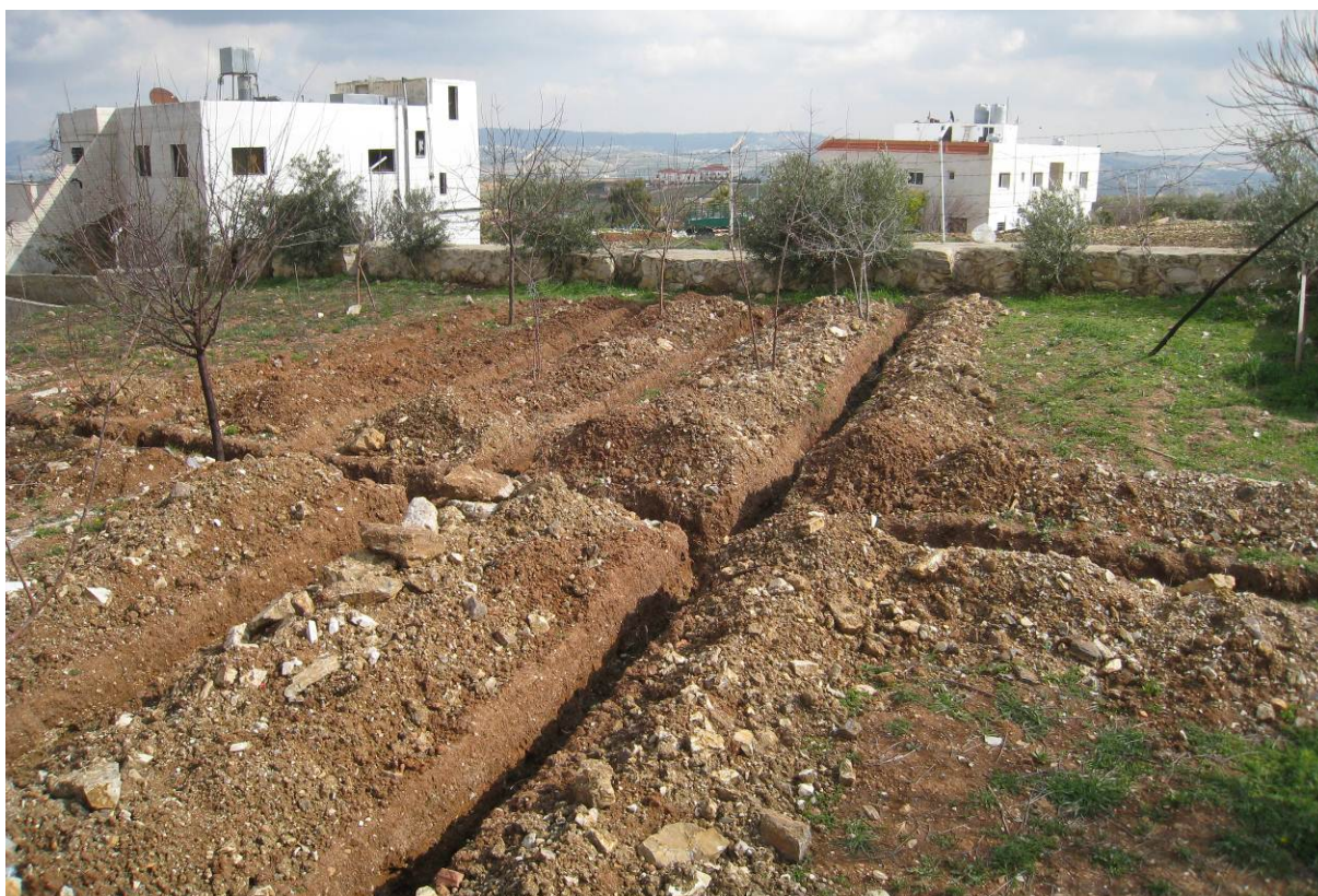
Figure 5: Excavation of the irrigation trenches at Mr Hiyari's house
