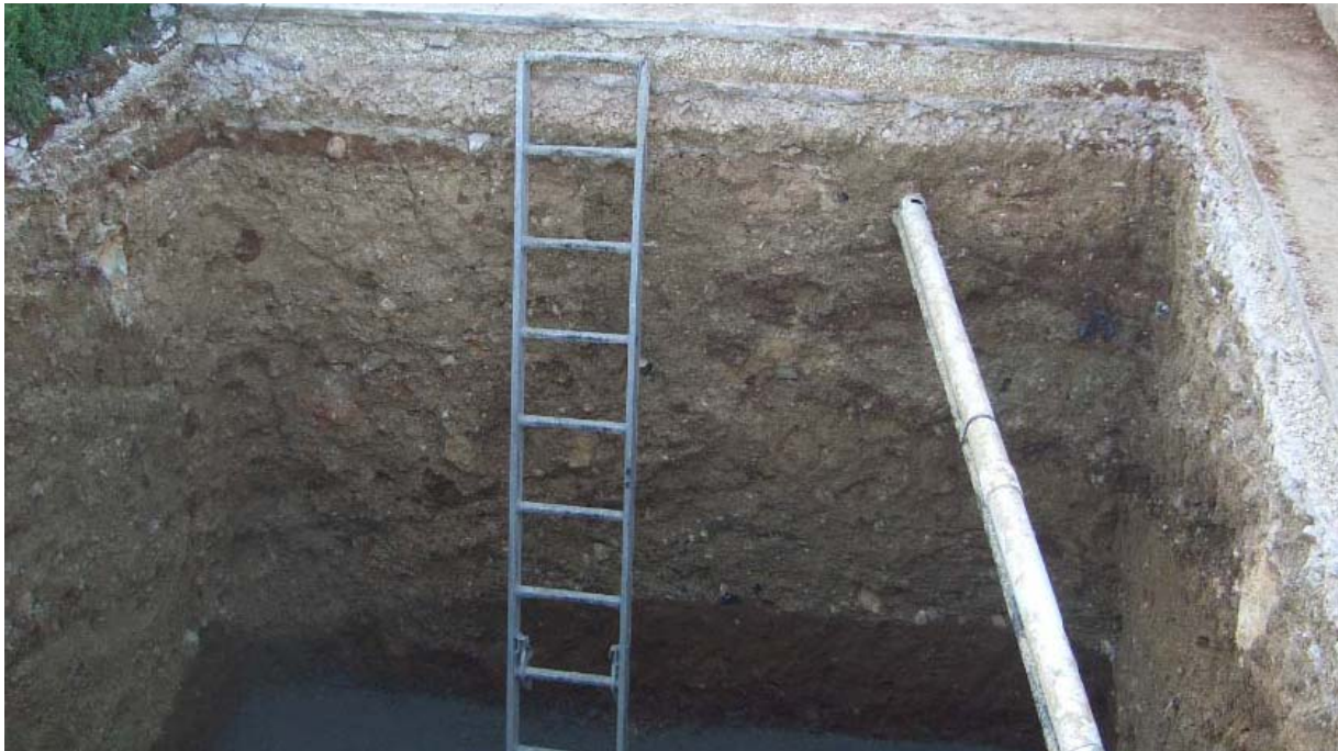
Figure 11: Excavation of the pit for the Modified Septic Tank.
