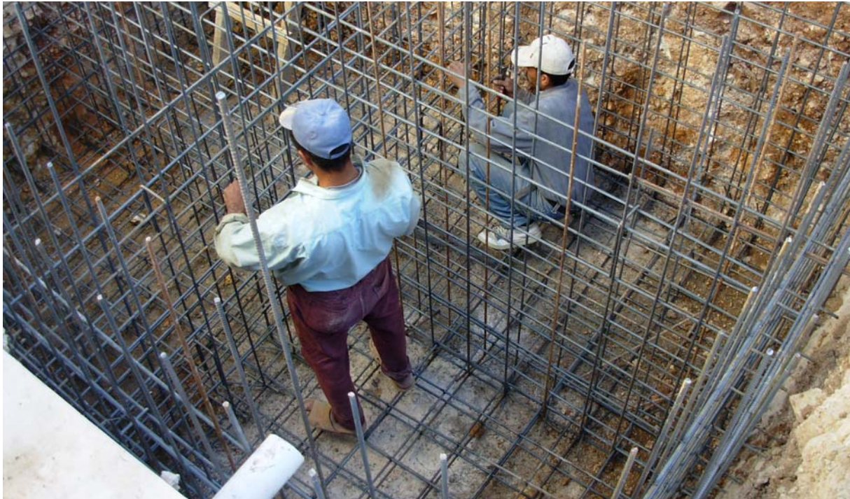
Figure 23: Installation of the reinforcement steel for the Modified Septic Tank.
